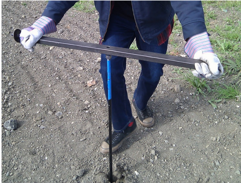
Ground anchor installation
