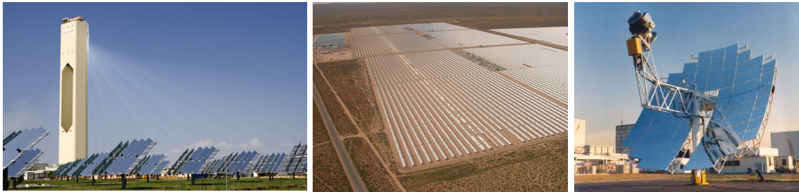
Examples of different types of CSP: tower, trough, and dish
